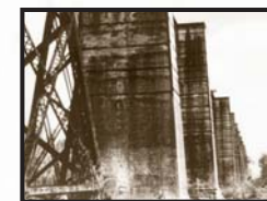
1914 bridge base (left) and original brick piers.
