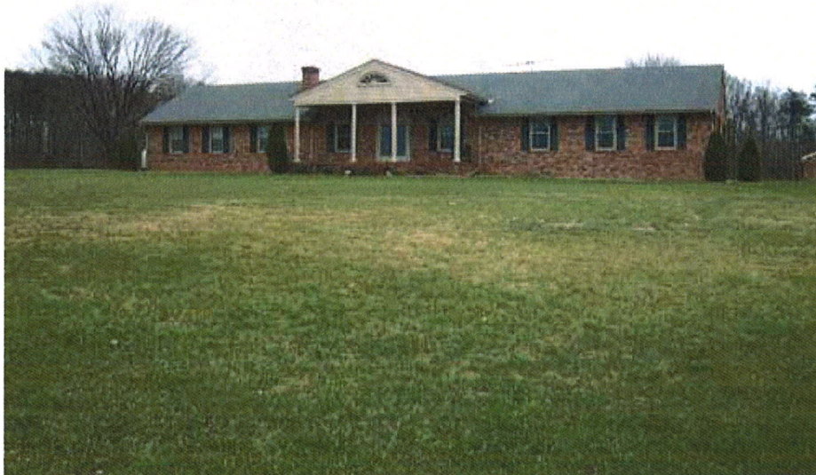
Front View of Residential Dwelling
