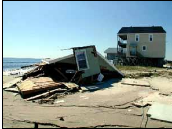
Hurricane Floyd brought a devastating 15 feet of storm surge that damaged or destroyed hundreds of houses along the ocean front of Long Beach on Oak Island, North Carolina in September 1999. A prime example of successful hazard mitigation can be seen in the photo above. The elevated home (right) survived while the older, ground-level block foundation of the home on the left was crushed. (Photo by Dave Gatley/FEMA News Photo)
