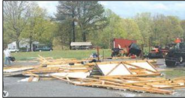
At least one confirmed tornado struck Lunenburg County on April 16, 2010. Areas north of Victoria were hit, with several houses and some other buildings receiving damage. Pictured above is tornado damage in and around the Victoria Golf Club. (Photo courtesy Kenbridge-Victoria Dispatch )
