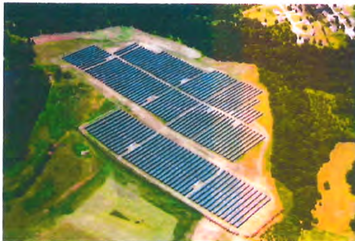
Figure 1: Utility-scale solar facility (5 MW AC ) located in Catawba County. Source: Strata Solar
