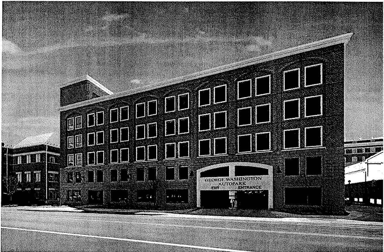
The 530-space, fully automated George Washington Autopark deck in Winchester was built using a public-private partnership. Photo by Eric Taylor Photography.
