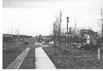
Example of buildings setback from highway
