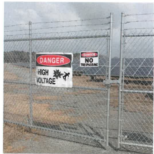
Figure 1. Perimeter Fence with Warning Signs
