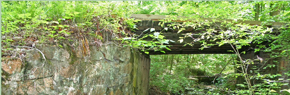
Prince Edward-Gallion State Forest (Photo Source: Virginia Department of Forestry)
